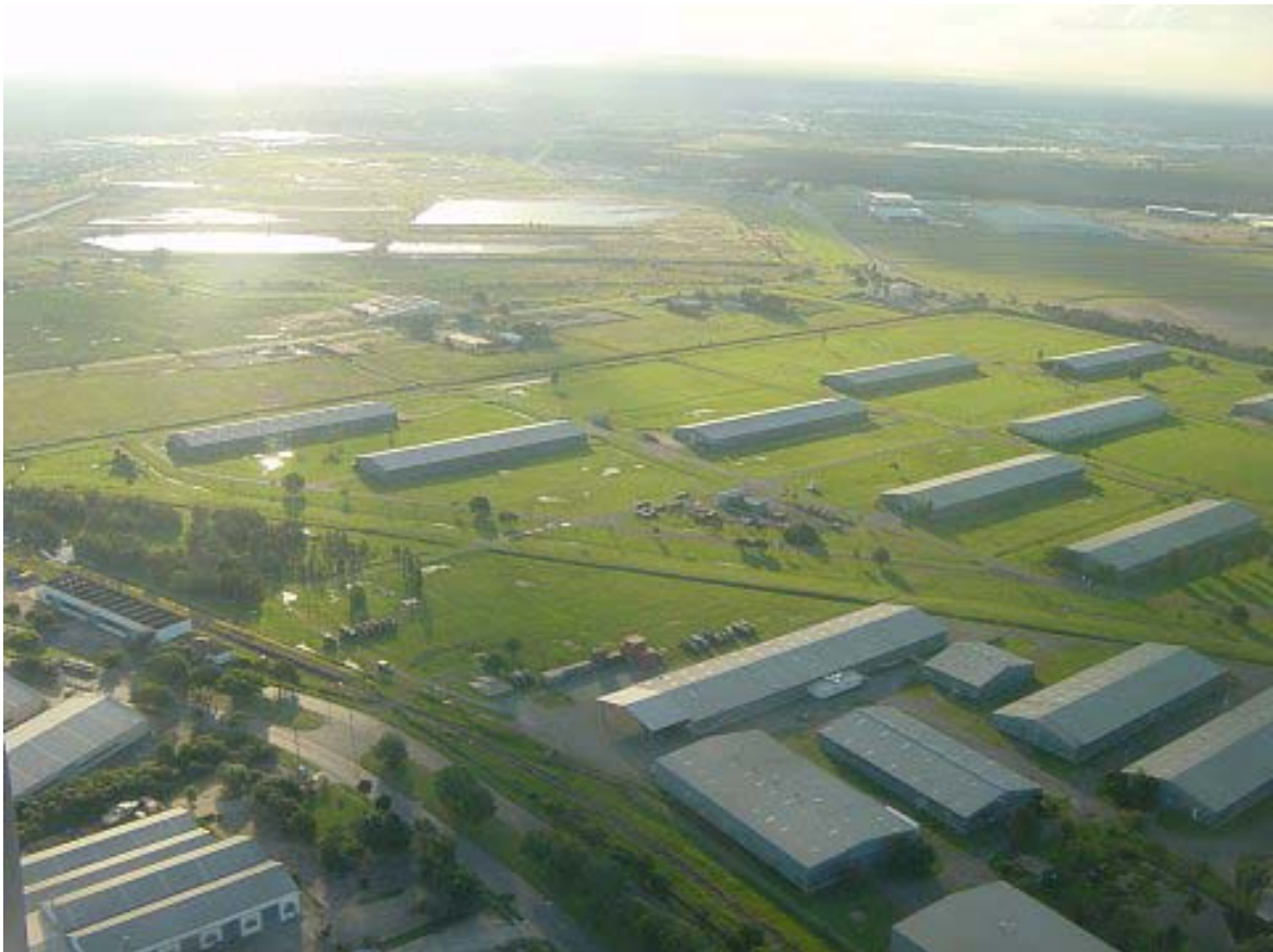
Photograph 2. Meeandah in June 2003.
