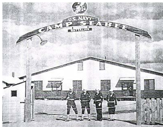
Photograph 6. A Picture of the entrance to Camp Seabee which is located in the centre right of the above photograph.
