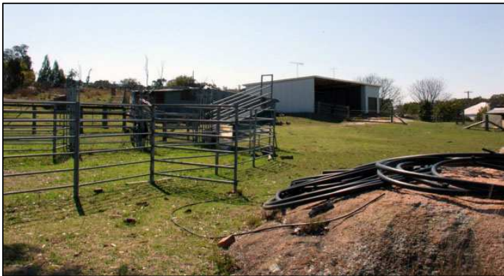
Figure 25: Carrels and sheds associated with the complex.
