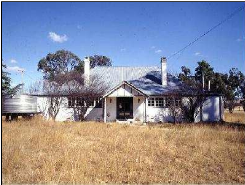
Figure 5: The Ballandean Homestead was the first substantial building erected in the Severn River district. (Courtesy EPA QPWS).
