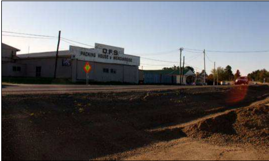
Figure 31: NW view of Q.F.S Packing House and Merchandise from the original site of the Applethorpe Railway Station.
