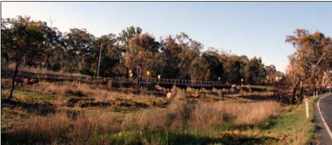
Figure 32: NNW view of Glen Aplin Rail Bridge.
