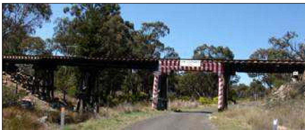
Figure 29: E facing view of timber rail bridge.
