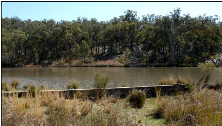
Figure 26: The dam with the cement weir in the foreground.
