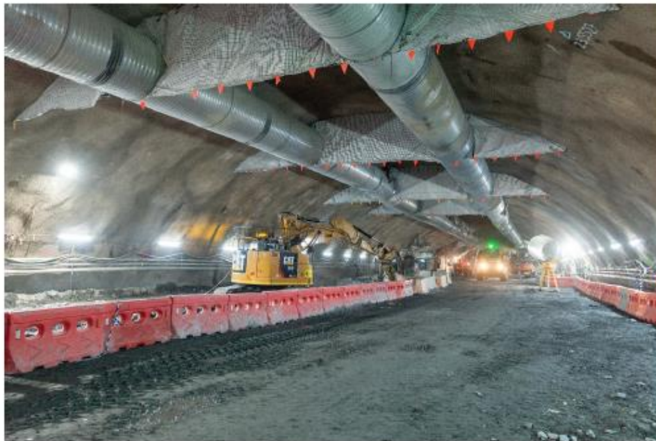
Image: Station cavern excavation at the Roma Street construction site
