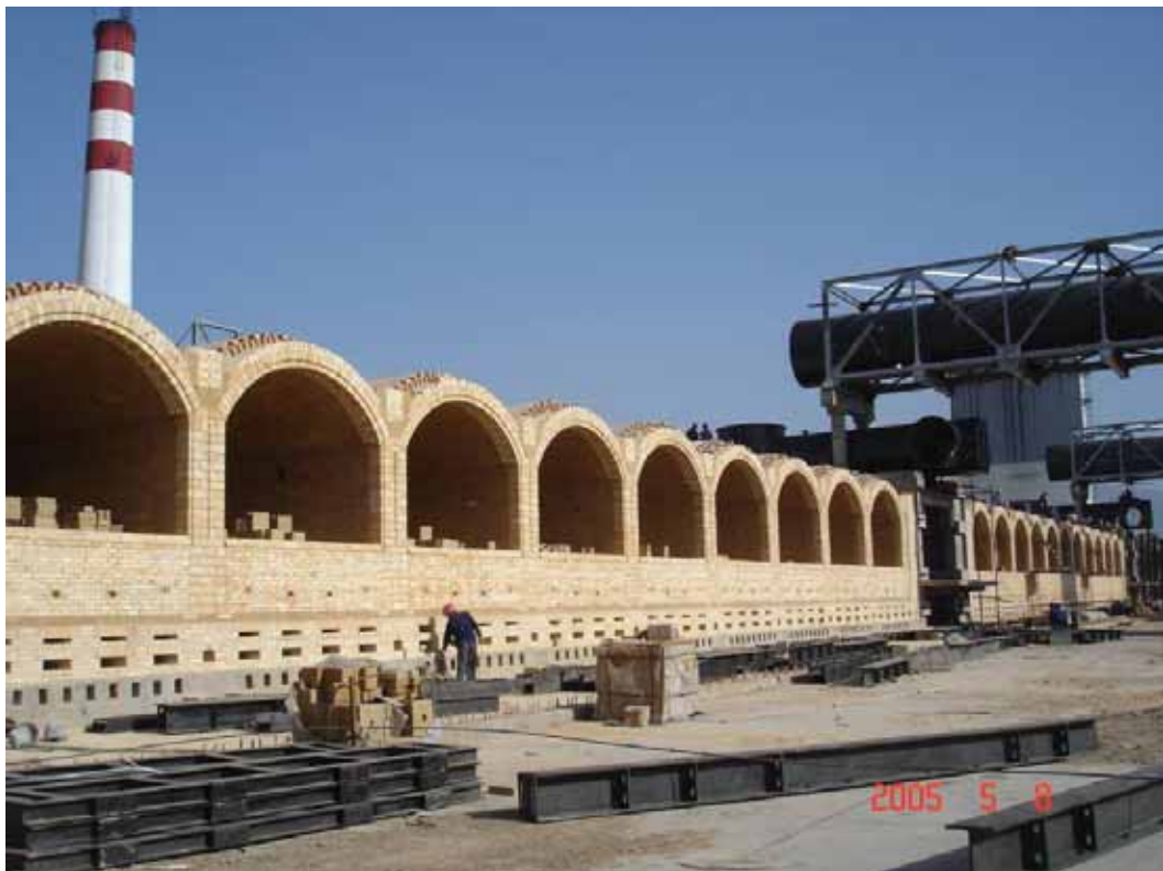
Plate 2.8 Coke Oven Construction in China
