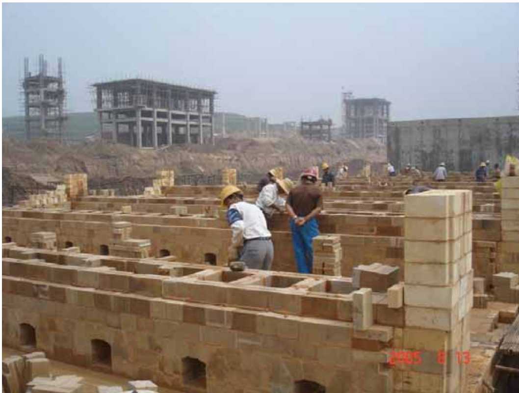
Plate 2.8 Coke Oven Construction in China
