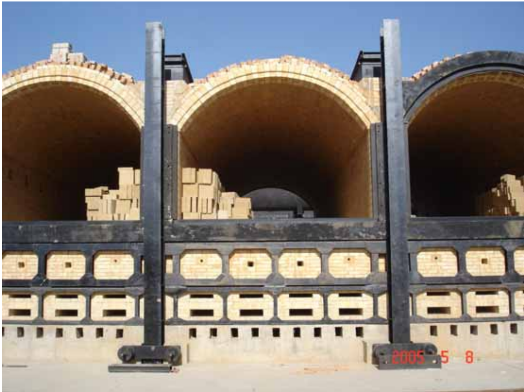
Plate 2.5 Example of the Construction of Coke Ovens
