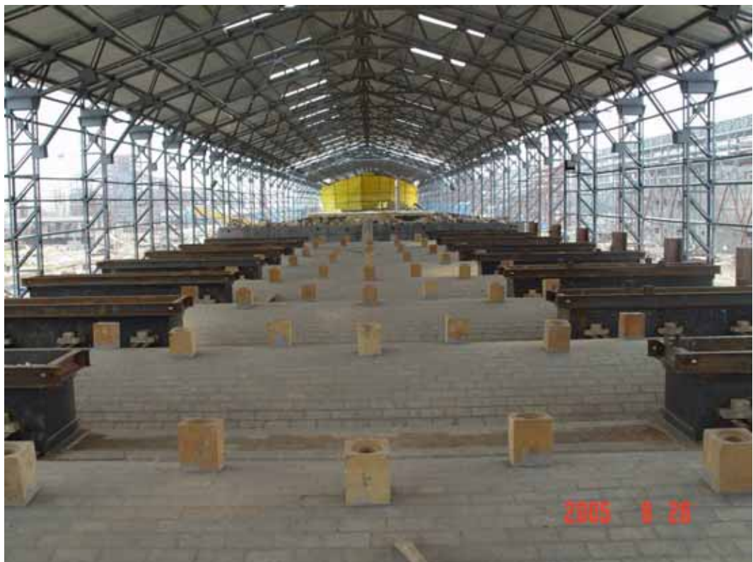
Plate 2.5 Example of the Construction of Coke Ovens
