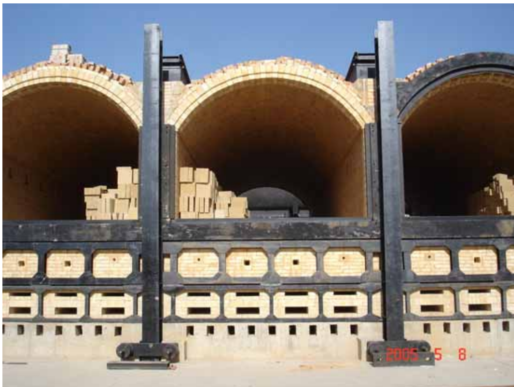
Plate 1.1 Example of Bee Hive Shaped Coke Ovens under Construction
