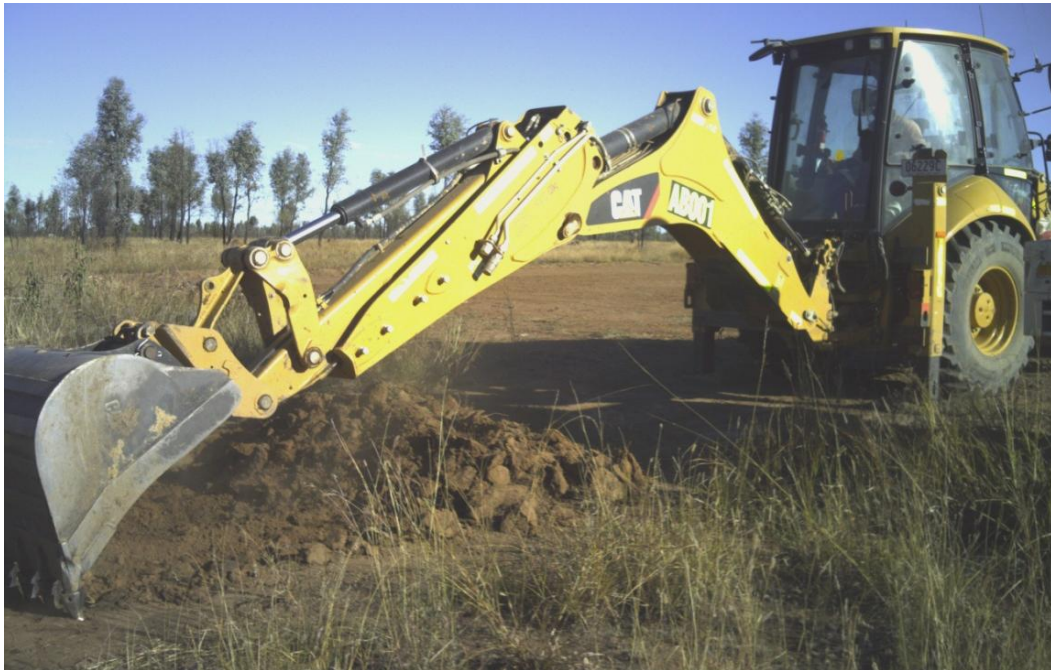
Figure 1: Excavation of surface layer assumed to be consistent with “topsoil” that would be stripped for rehabilitation.
