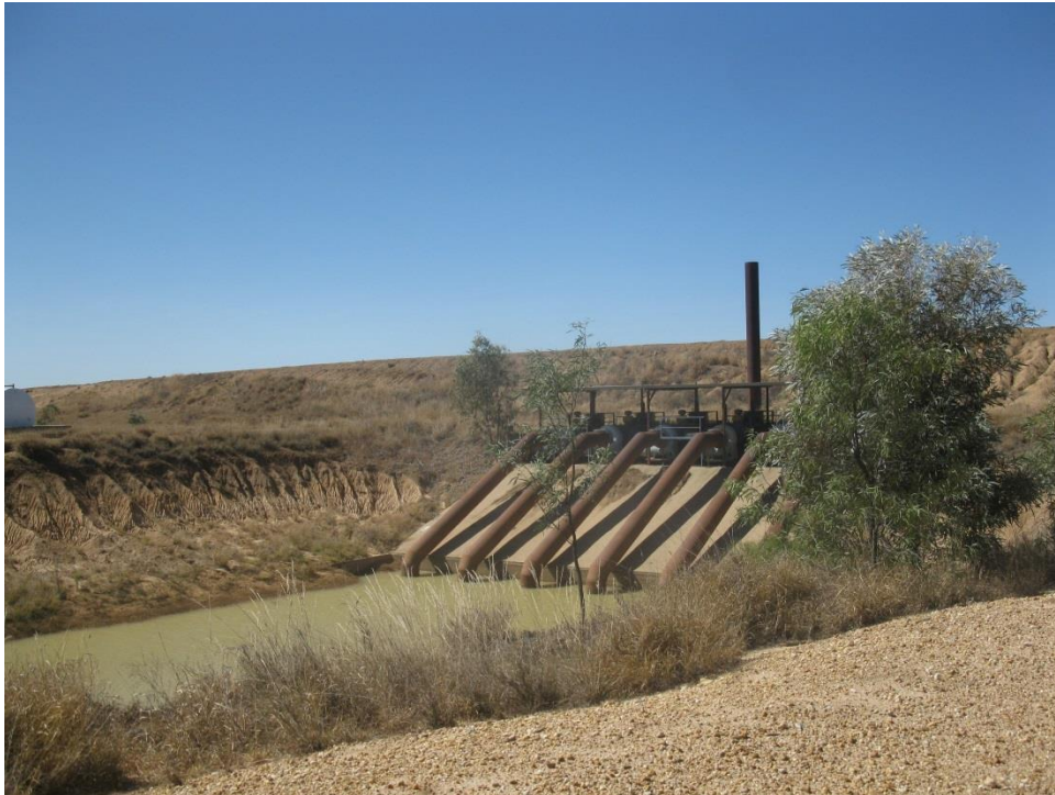
Photograph 10 – Existing diesel pumps within gravity diversion (ring tank in background)
