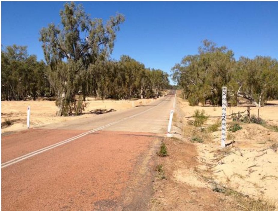
Figure 5.12: Cape River Crossing Causeway and Bridge, photo taking looking south from the northern bank on the Gregory Developmental Road. Note river height marker in the foreground. The bridge section is in the background before the rise on the southern bank.
