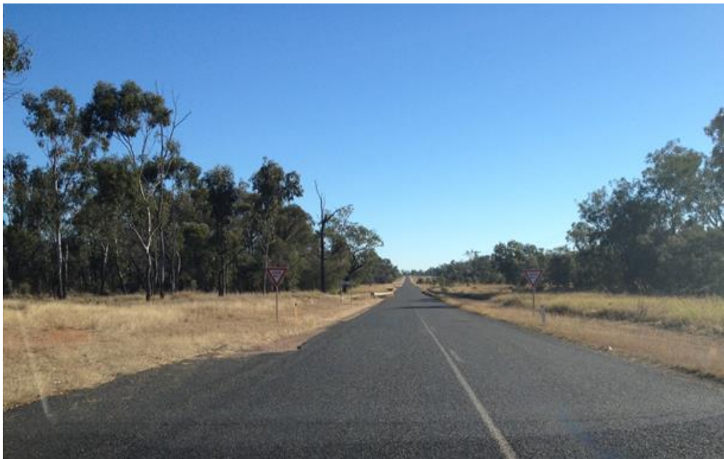
Figure 5.9: Miclere Creek Bridge (Gregory Developmental Road) – photo taken looking north. Note Give-Way signage, narrow bridge in background and wider pavement for stopping away from the bridge section
