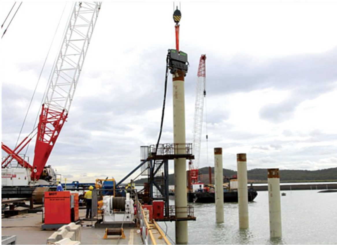
Photo C3-3 Example of a pile driving equipment.
