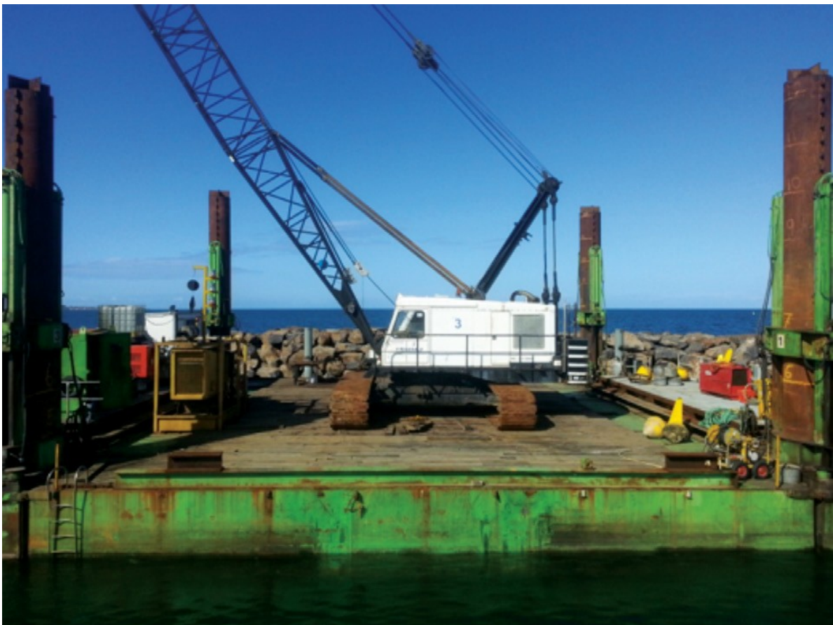
Photo C3-4 Example of a work barge.
