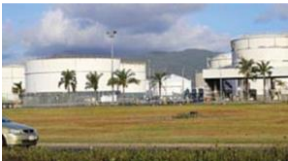
View towards fuel tanks from Kenny Street (ARUP)
