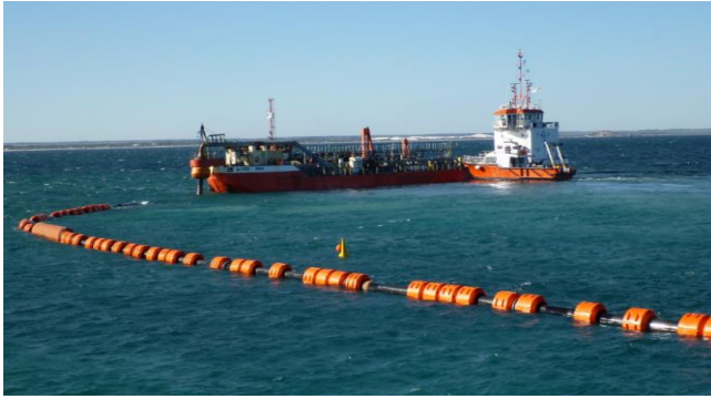
Photo A3-5 TSHD connection to floating pipeline.
