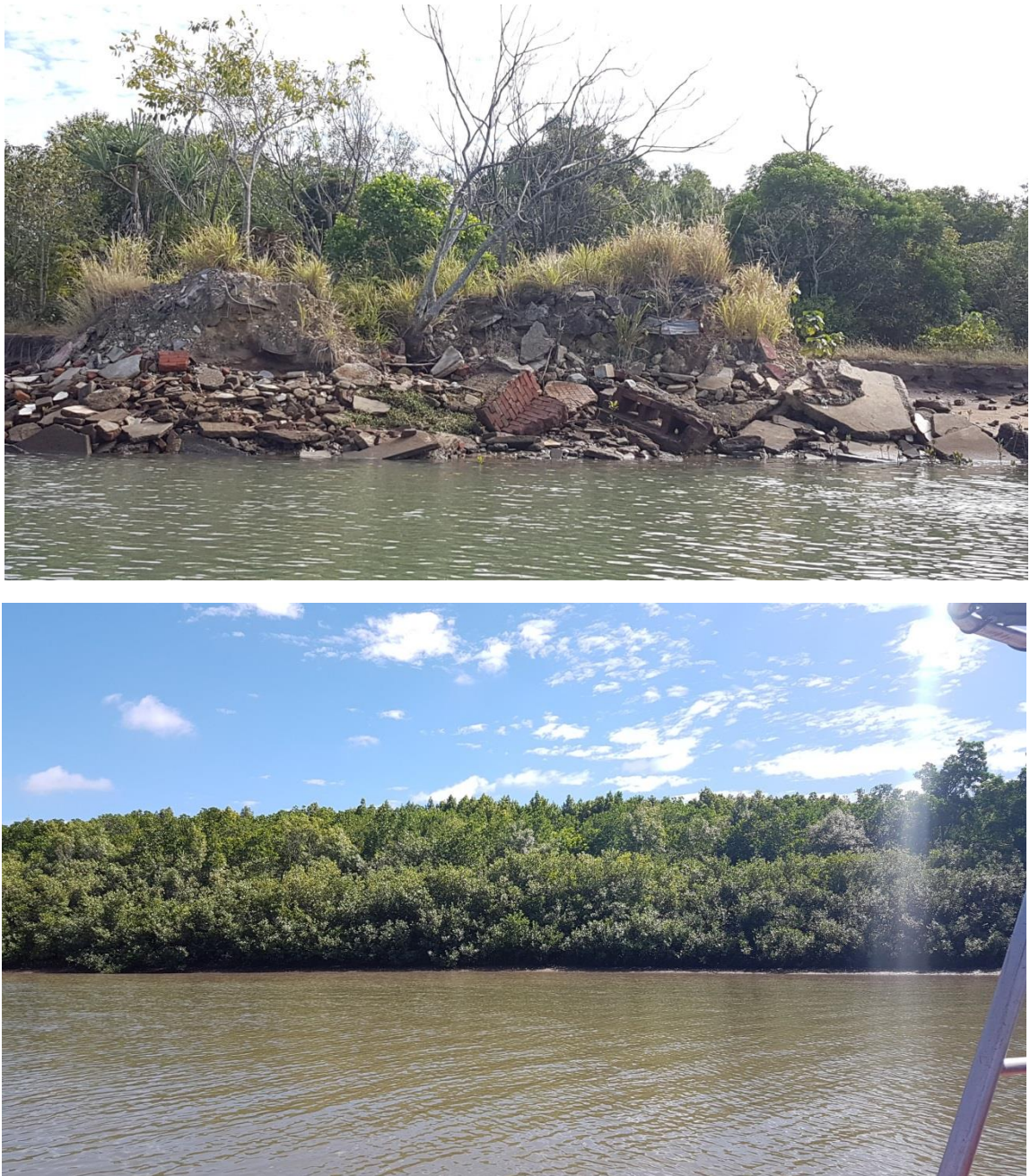
Figure 3-31 Armoring of the left bank with materials of opportunity in the downstream reaches (above); healthy mixed mangrove community in the mid section of the Barron River, DLB (below)
