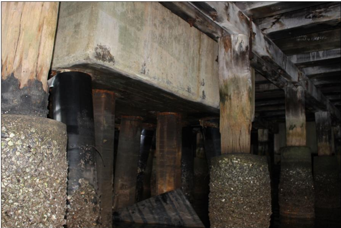
Timber substructure of wharf and concrete structure.
