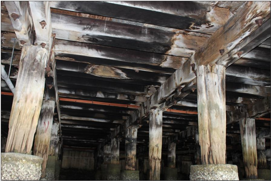
Timber substructure of wharf.
