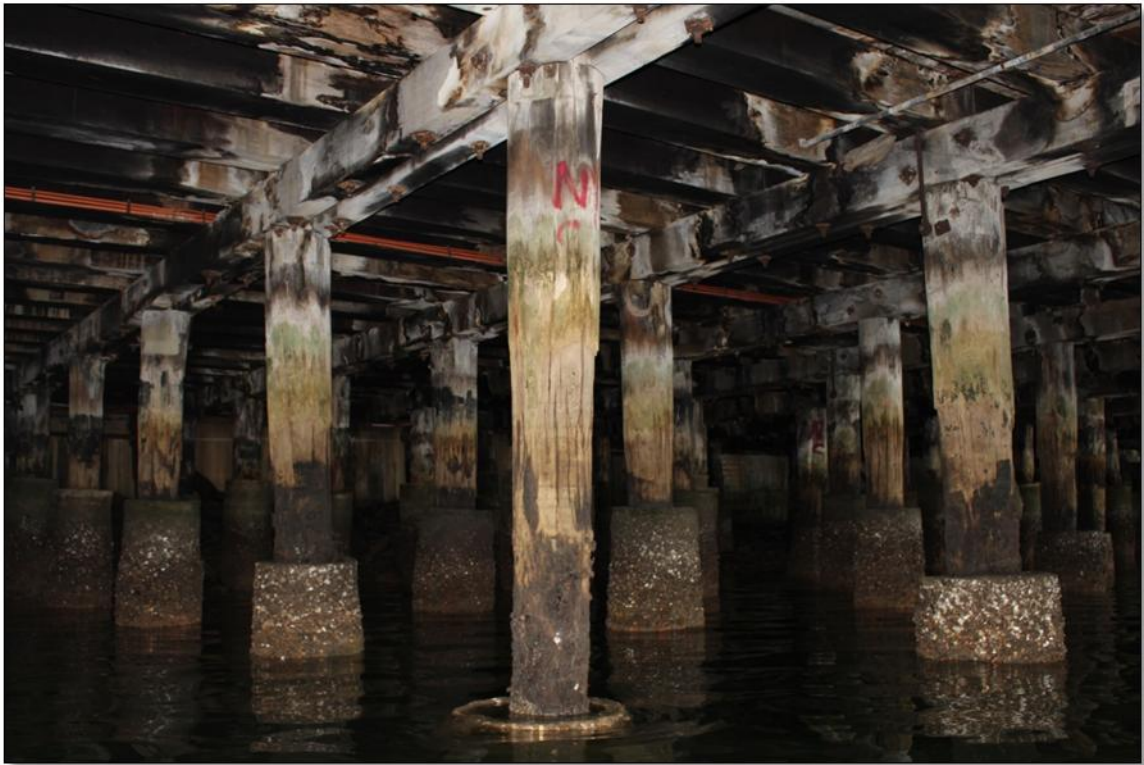
Top portion of concrete sleeve at same height of water level.
