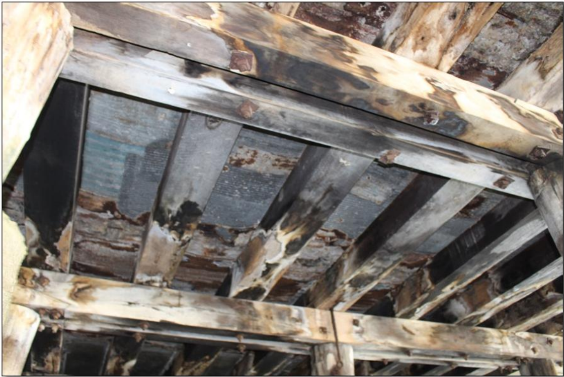
Staining on headstock surface.
