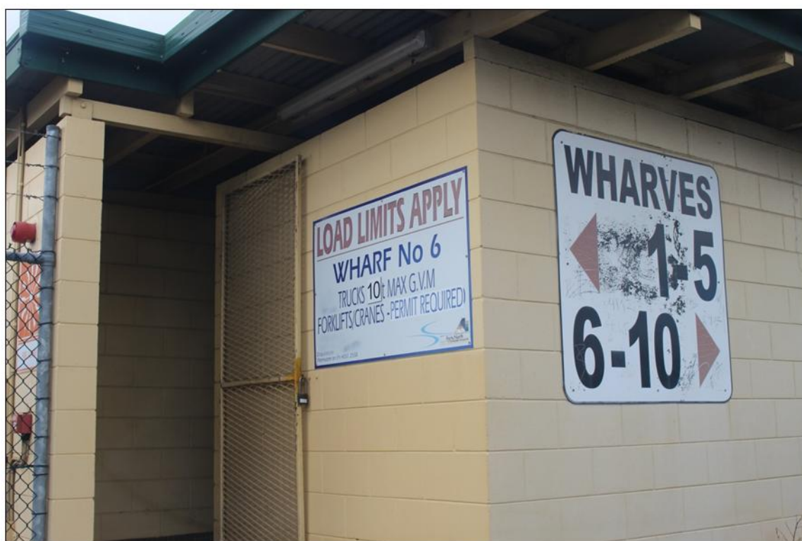
Current load limit to Wharf 6.
