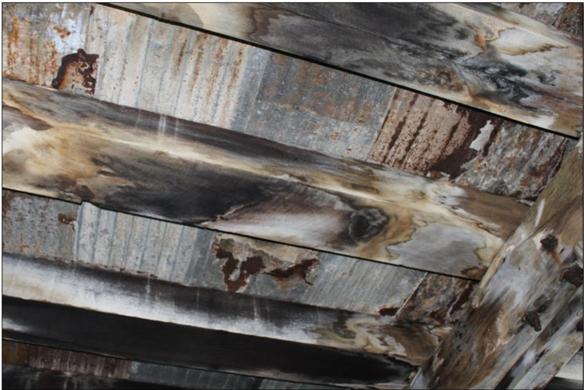
Galvanised steel formwork over timber girders.
