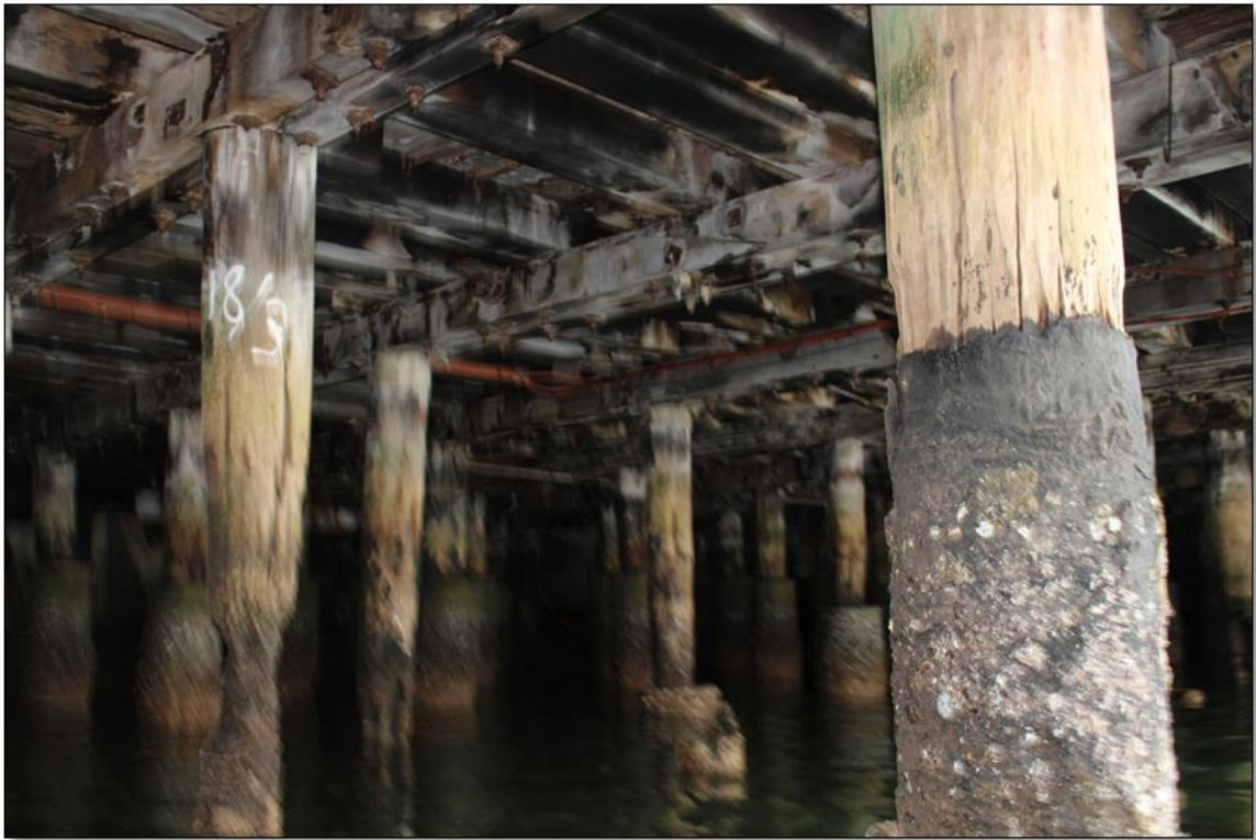
Pile wrapped with epoxy coating.
