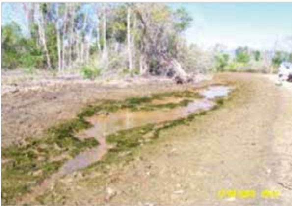
A road drain at East Trinity in 2003 and 2010 (source: DSITIA)
