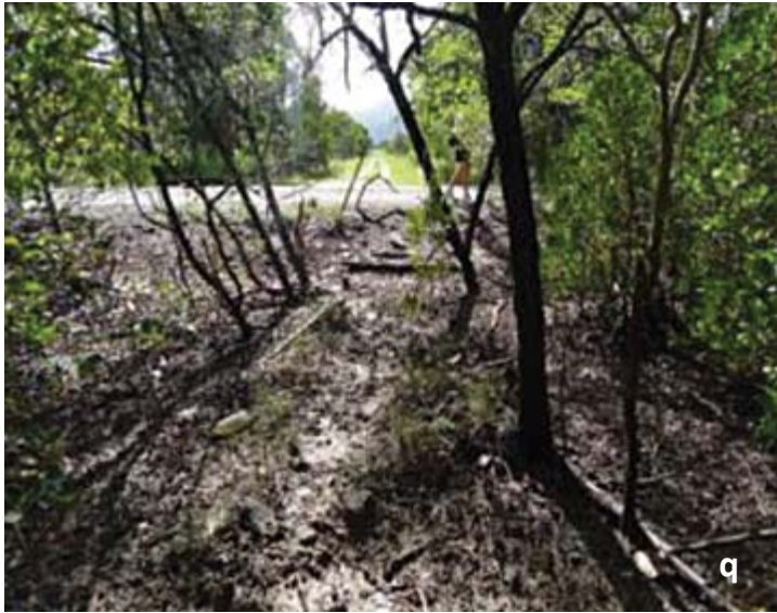
Figure B13.8q-s Tramway. View to west from bund wall.
