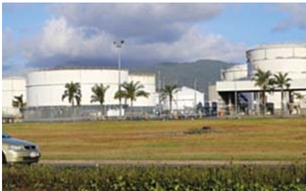
View towards fuel tanks from Kenny Street
