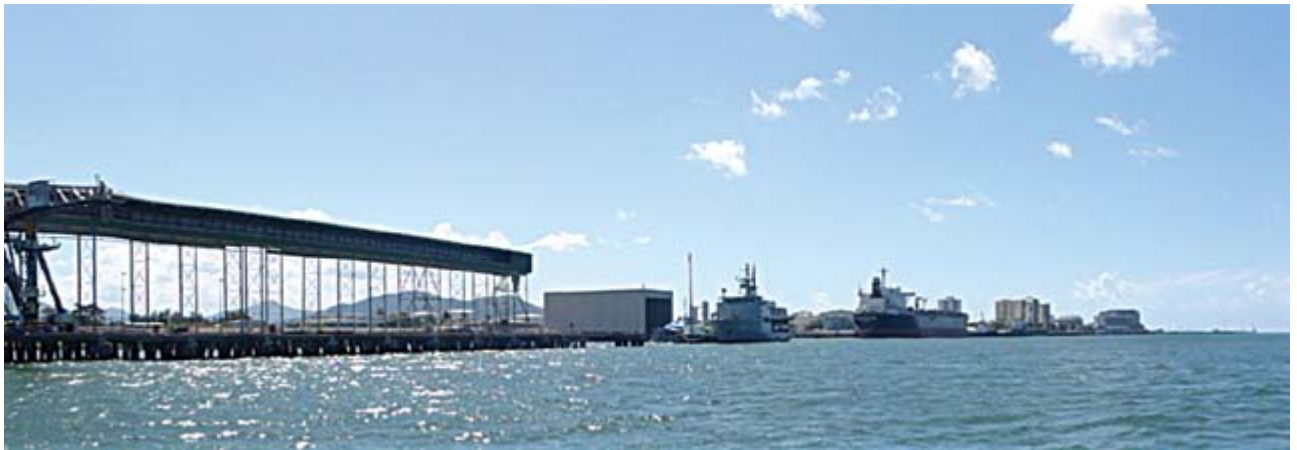
Figure B1.4.1a Inner Port – view northwards from Wharf 12 (Sugar Wharf)
