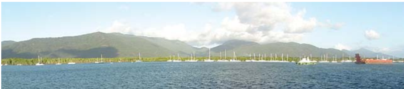
Figure B1.4.5a Pile Moorings – Eastern Side of Trinity Inlet
