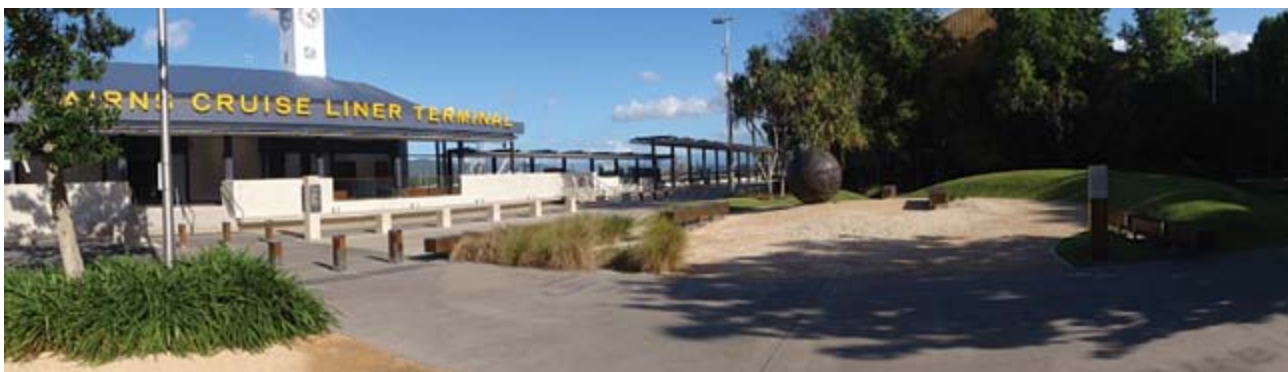
Figure B1.5.1a Cairns Cruise Liner Terminal
