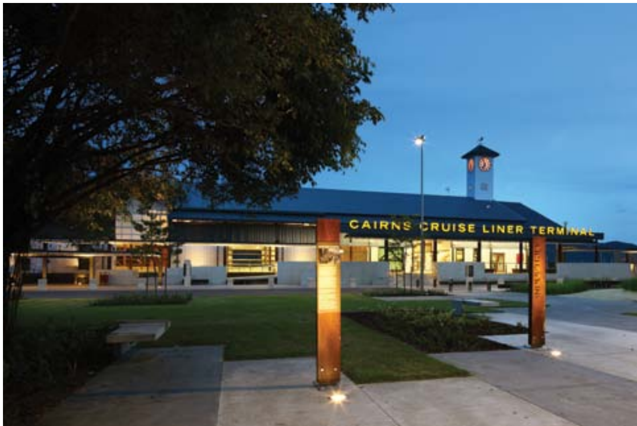
Figure A4.2.5.1a Landward view of the Cruise Terminal (Shed 3)
