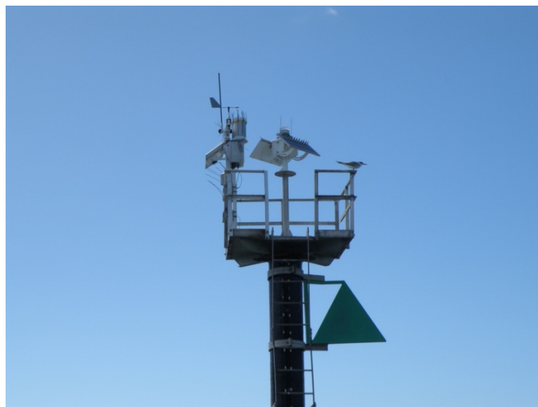
Figure A-9 Envirodata Maestro Weather Station Installation at Site 5 (Beacon C11)
