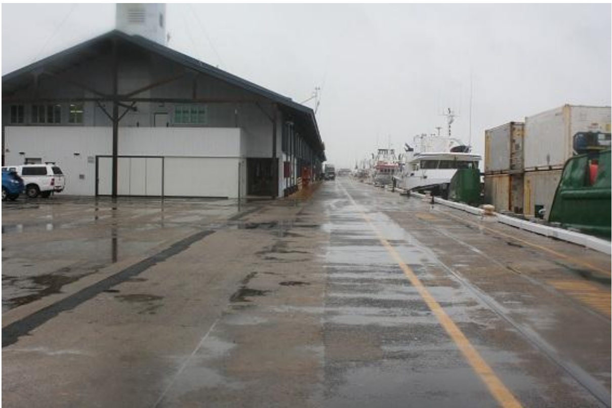
Figure 21. View northwards of wharves 3 and 2, with the Wharf 3 Shed on the left.
