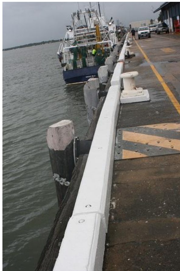
Figure 23. The wharf edge, showing concrete kerbing blocks and cone-mounted fender piles.
