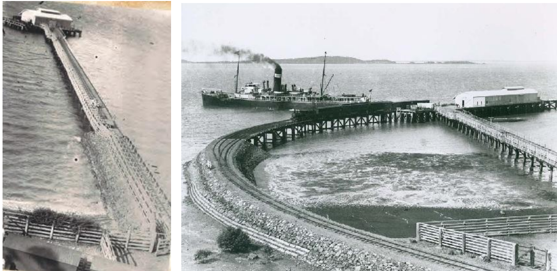
Figure 10. Auckland Point Jetty circa 1908, prior to its extension in concrete (left) (Source: Gladstone Regional Art Gallery and Museum) and (right) in the 1920s after its extension (note the railway connection).(Source: QSL)
