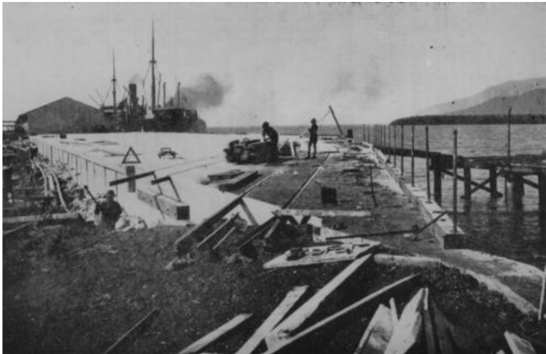
Figure 16. Construction of Wharf 5 at Cairns, circa 1920s. The rail tracks are set into the deck of the wharf and the future site of Wharf 6 is on the right. (Source: SLQ #186298)
