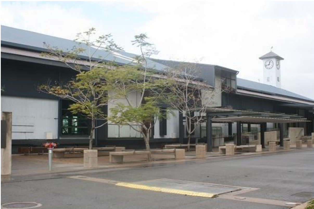
Figure 25. The Wharf street frontage of the Wharf 3 Shed; note the skillion section in the roofline which is a remnant of the former conveyor connection from White's Shed.
