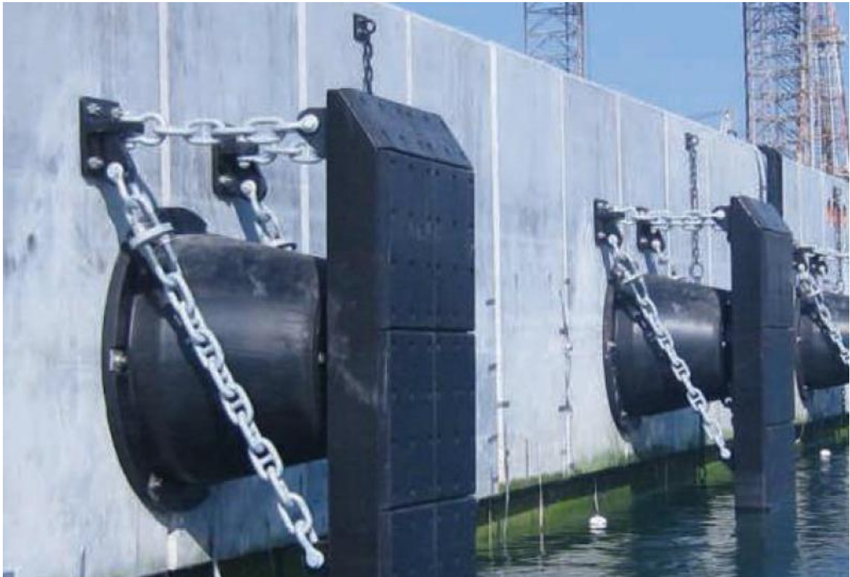
Figure 33. Indicative view of an installation of ‘Super-Cone Fenders’ (at Bahrain) (Source: Ports North).
