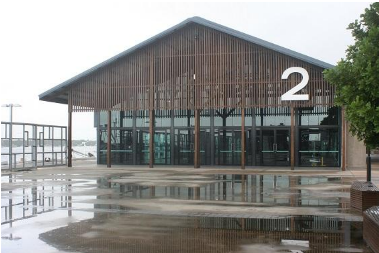
Figure 26. The redeveloped north end of Wharf Shed 2, with glazed wall panels and timber screen.
