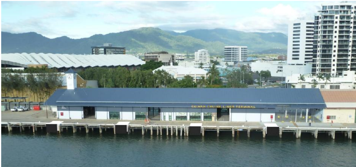
Figure 32. Generated image of the proposed new berthing dolphins inserted into the wharf deck, visible as white/black patches along the front of the wharf. Note: The white and black in the image is to assist the reader only. The actual finish would be grey concrete similar in appearance to the historic fabric. (Source: Ports North)
