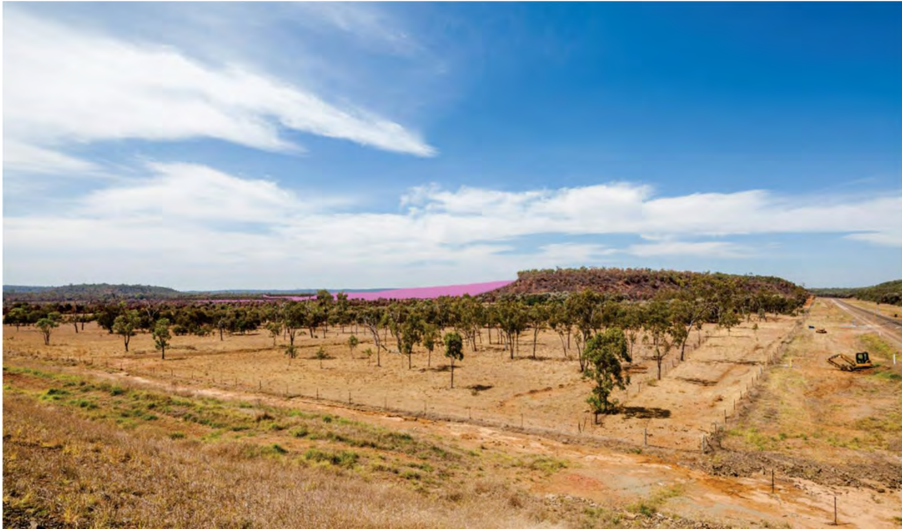
Figure 25-4 Photomontage 1 b Collinsville-Elphinstone Road (from Railway Bridge) Worst Case Scenario Visual Envelope
