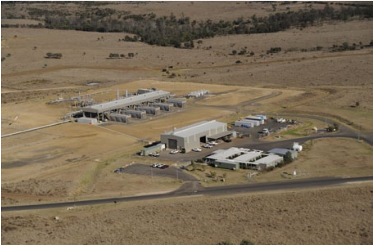
Figure 4 Australia Pacific LNG's operating gas processing facility at Spring Gully
