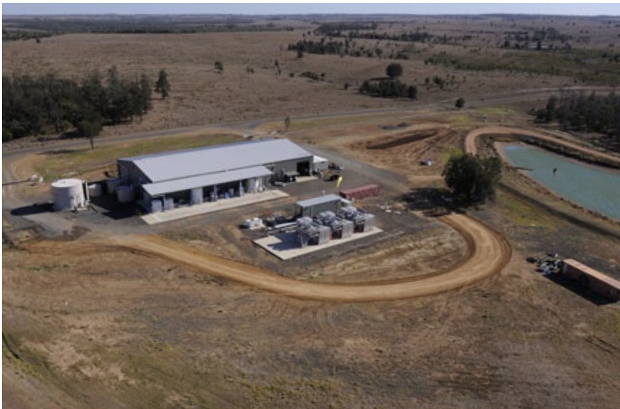
Figure 5 Australia Pacific LNG's operating water treatment facility at Spring Gully
