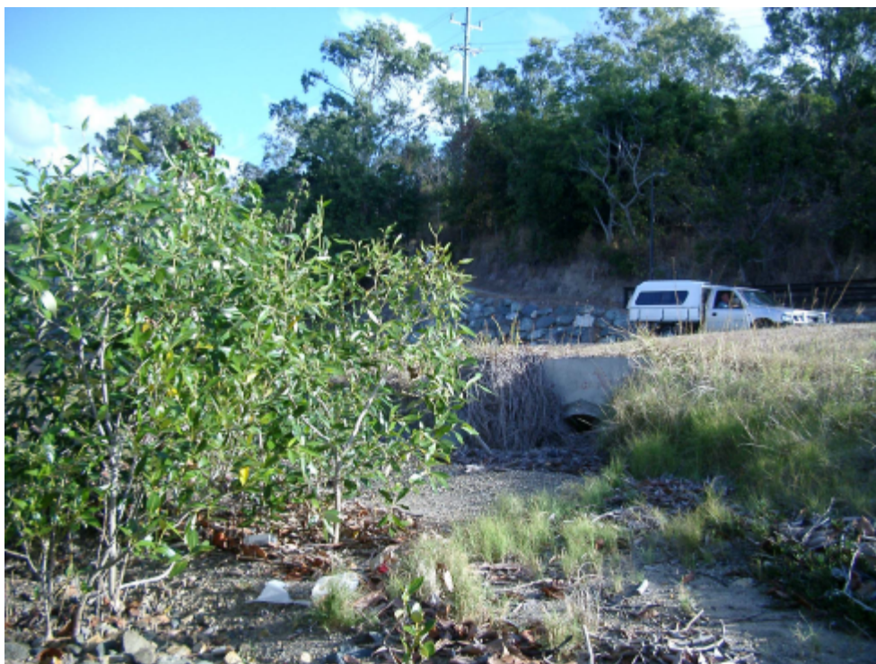
■ Figure 8-7 Stormwater Discharges into the Mangroves at 100 m intervals along the Proserpine – Shute Harbour Road
