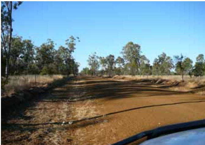
Plate 9-2. A wider, formed earth, section of Nathan Road north of Cockatoo Creek
