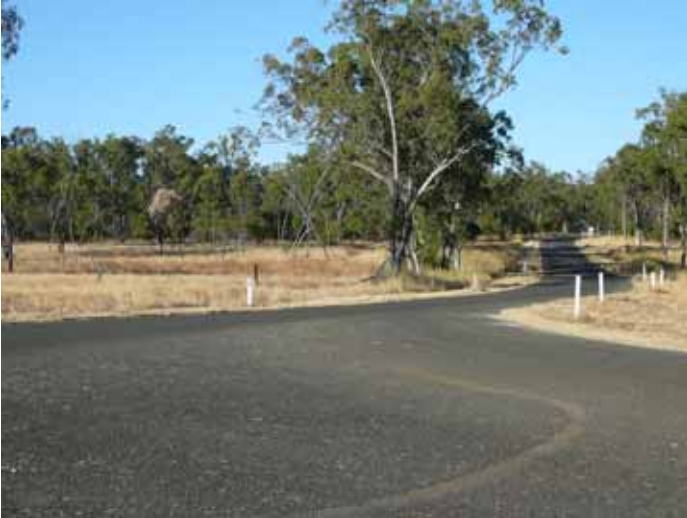
Plate 9-4. A single lane bitumen sealed and paved part of the northern section of Nathan Road at the intersection with the road to Eidsvold via Dearne just north of Cockatoo Creek
