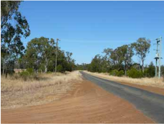
Plate 9-1. The southern, single lane, bitumen paved and sealed section of Nathan Road north of Roche Creek
