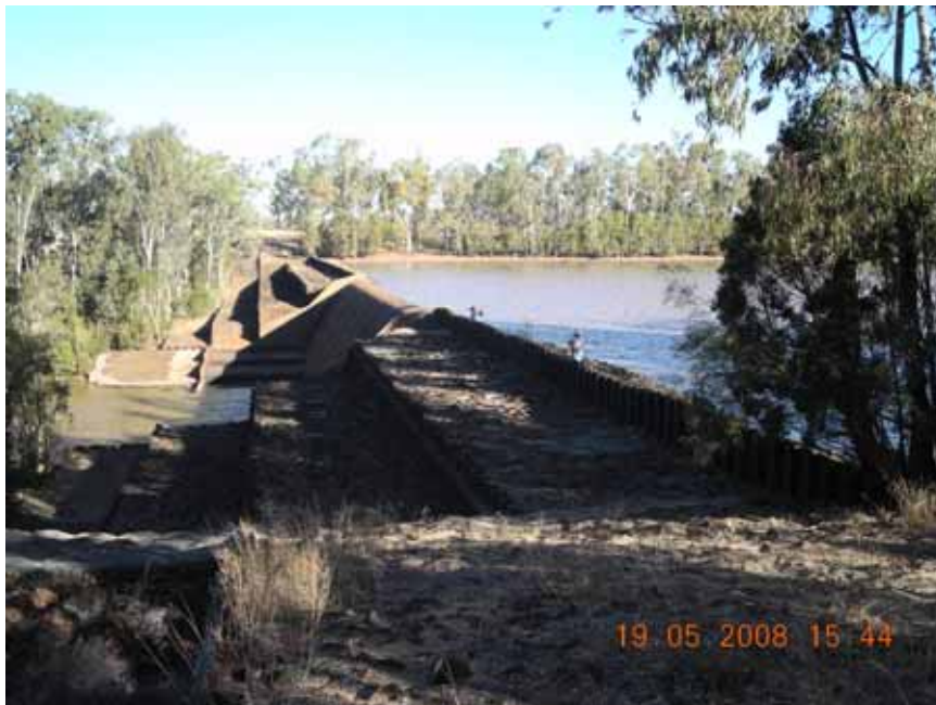
Plate 5-1. Glebe Weir showing central spillway crest flanked by stepped sheet pile abutments
