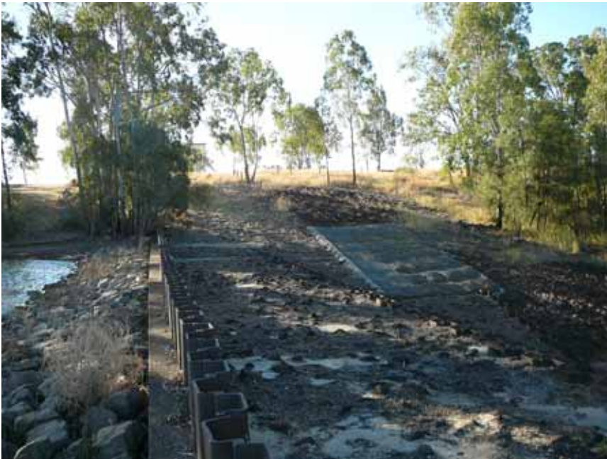
Plate 5-2. Left abutment of Glebe Weir showing rock pitching on upstream battered fill, downstream rockfilled mattresses, rip rap extending up the river bank and three rows of sheet piling
