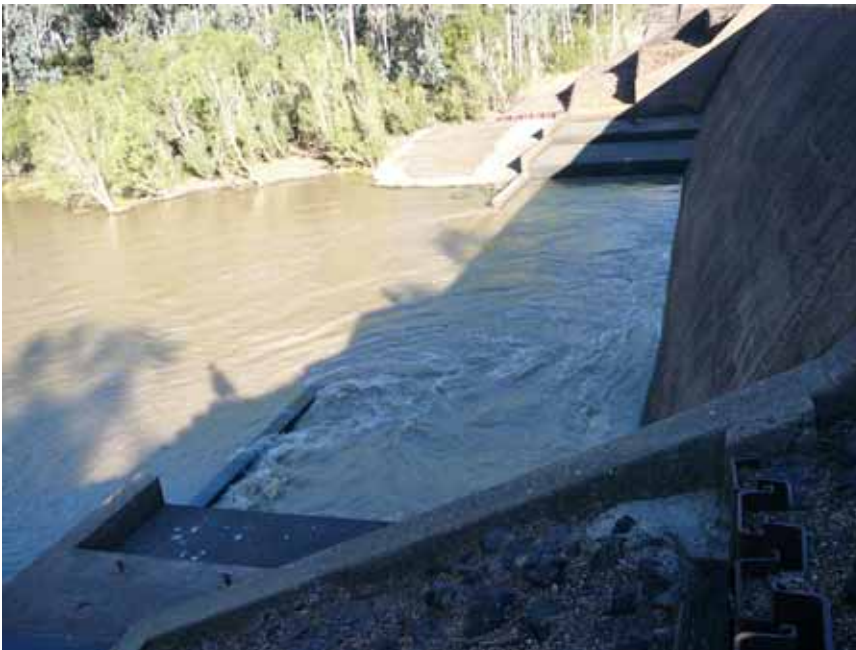
Plate 5-3. Releases from Glebe Weir discharging onto the apron downstream of the spillway with deck over valve pit in lower left
