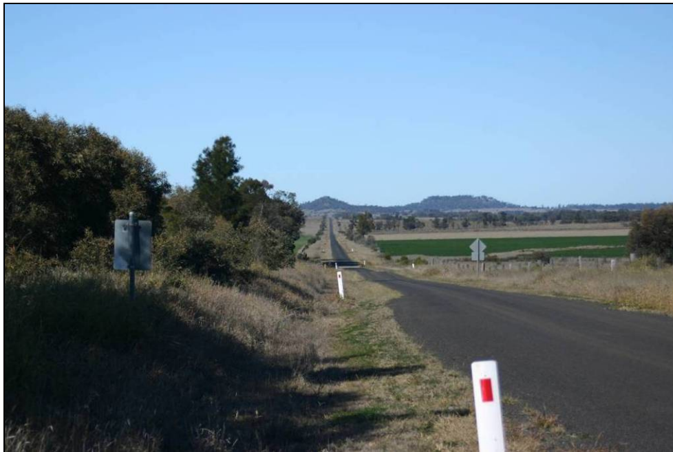
Figure 19-10: Linear strips of roadside vegetation are frequent along Peakes Road
