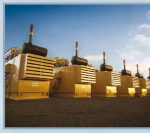
12MW gas-fired power station using methane extracted from XCQ's Oaky Creek Mine, QLD
