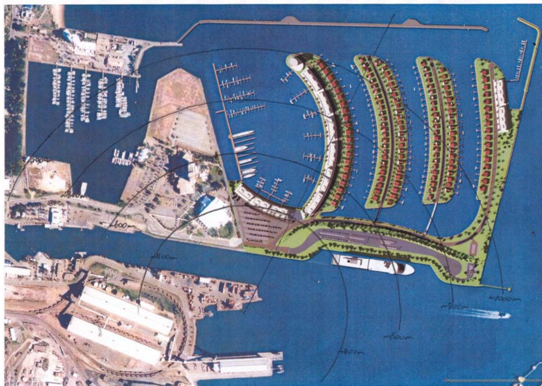
FIGURE 1: PROXIMITY OF BREAKWATER COVE RESIDENTIAL BUILDINGS TO BERTH 10
