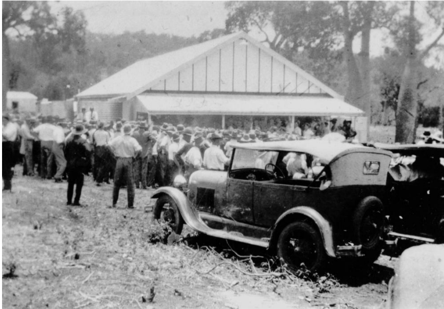
Figure L.3: Land sale at Golden Mile store, Cracow, Queensland. It took some time for the town of Cracow to be surveyed after gold was discovered, but lots sold briskly in the booming mining town (JOL ban00085)
