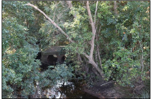
Plate 22. A dislodged culvert, in Six Mile Creek, north of the spillway will be removed with a crane.
