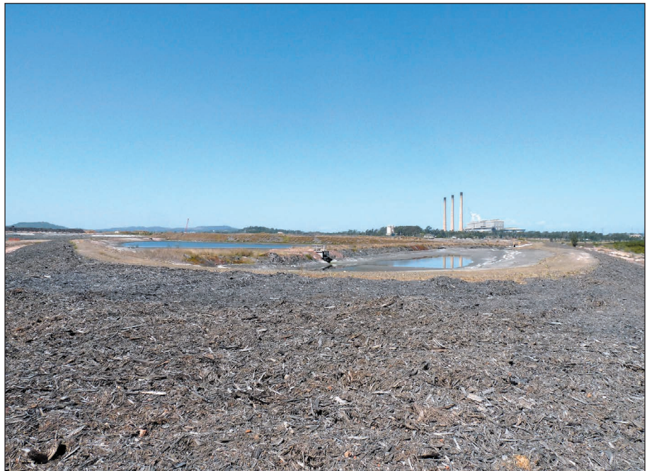
Plate 19.4 Clinton ash ponds (northern pond)
