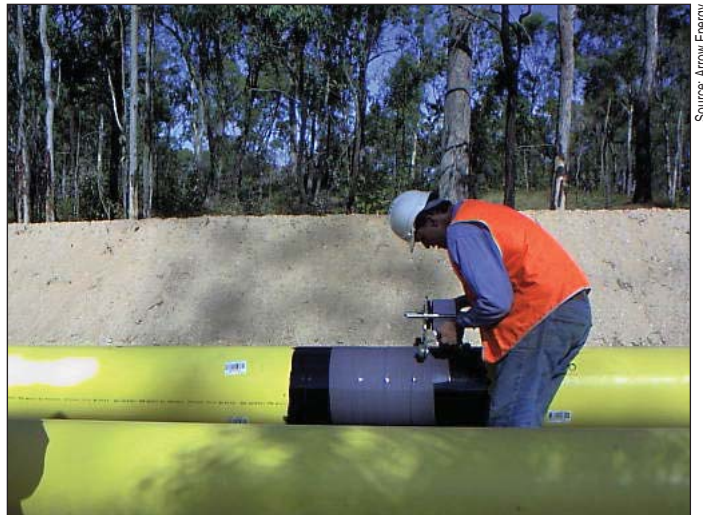
Plate 7.5 Coating and wrapping of the pipe joint
