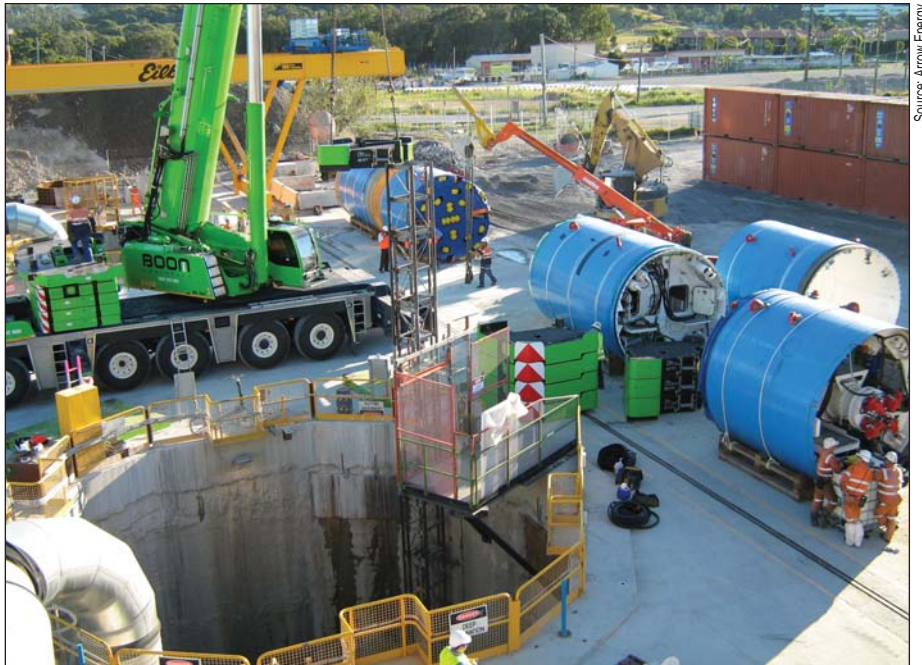
Plate 7.2 Typical launch shaft and TBM segments ready for lowering down shaft
