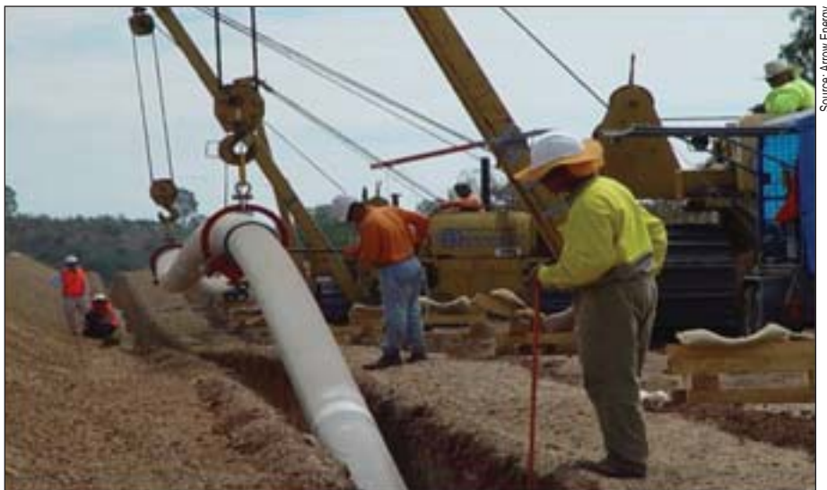
Plate 7.6 Pipeline being lowering into the trench
