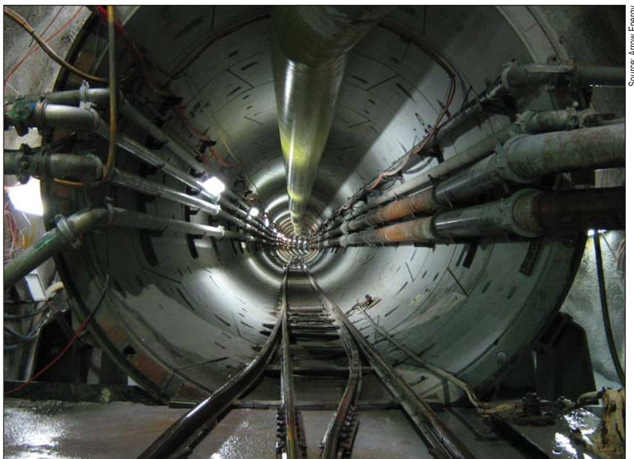
Plate 7.3 Typical TBM-bored concrete-segment-lined tunnel
