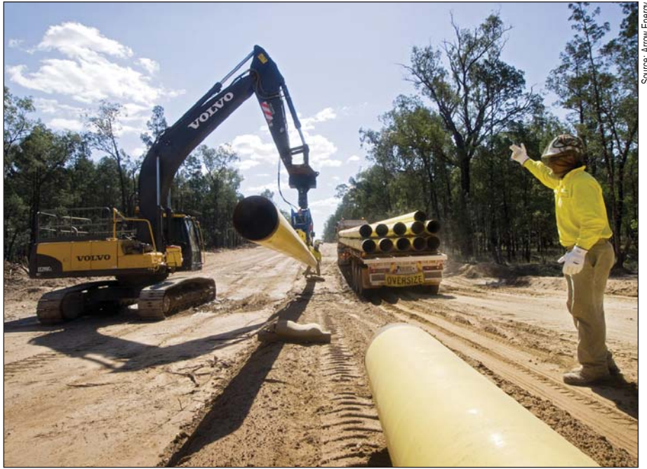
Plate 7.4 Pipeline stringing
