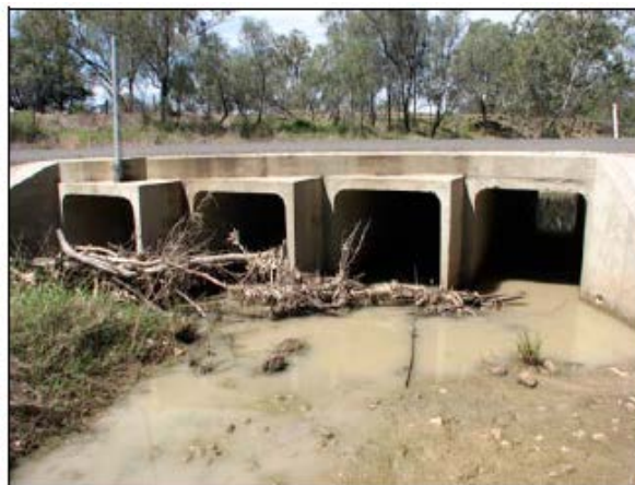
Plate 4-9 Obstructions upstream of the box culverts on Wallumbilla Creek likely to restrict the passage of aquatic fauna.
