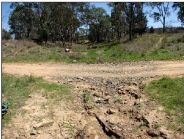
Plate 4-8 Unformed crossings act as a physical barrier to water flows and aquatic passage during periods of very low flow
