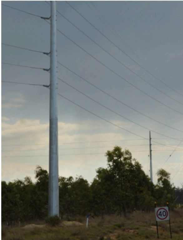
Plate 5-15 Current 33 kV above ground power lines
