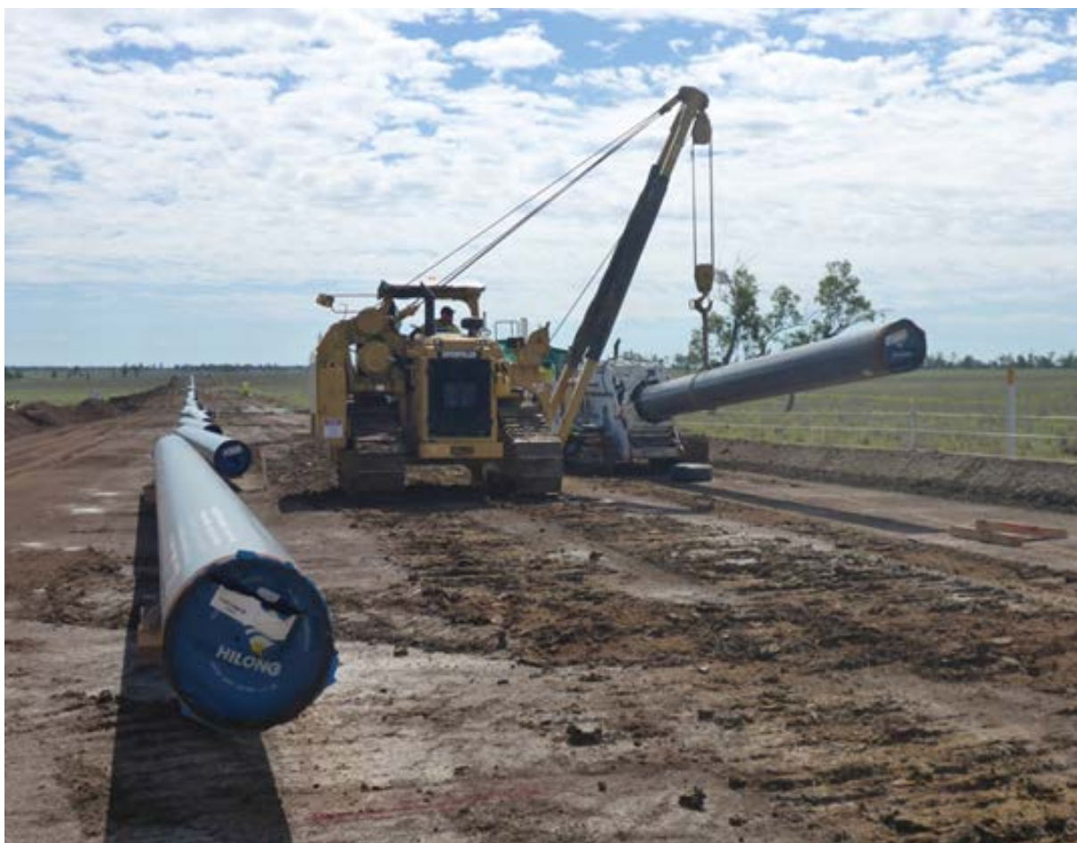
Plate 5-4 Construction of transmission pipeline
