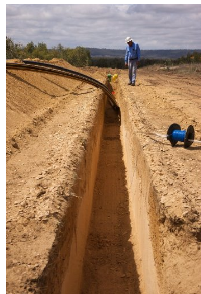
Plate 5-3 Construction of gathering lines
