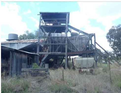
Photograph 12-1 Gantry and Hopper
