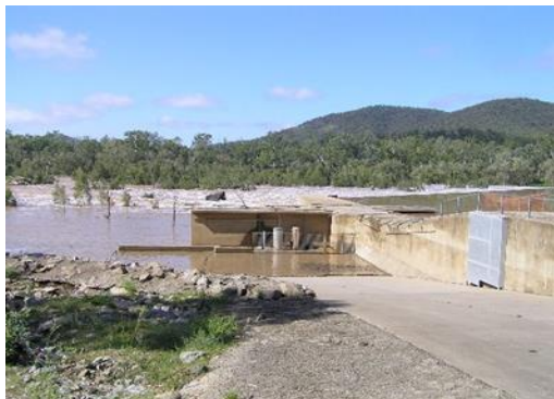
Left bank outlet works and fish lock
