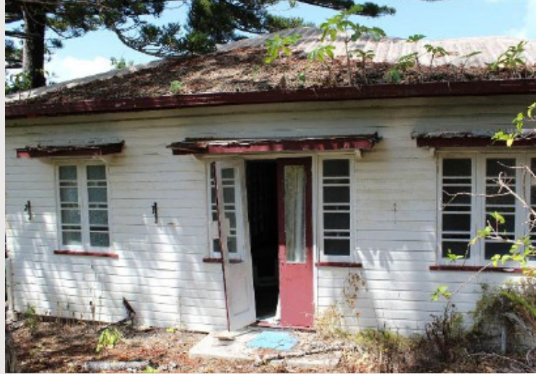
Figure 12-9. Northern elevation of Nicholson's Residence.
