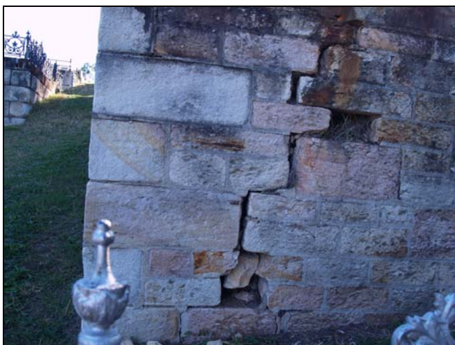
■ Figure 12-1. Badly cracked monumental masonry in Portion 13.
