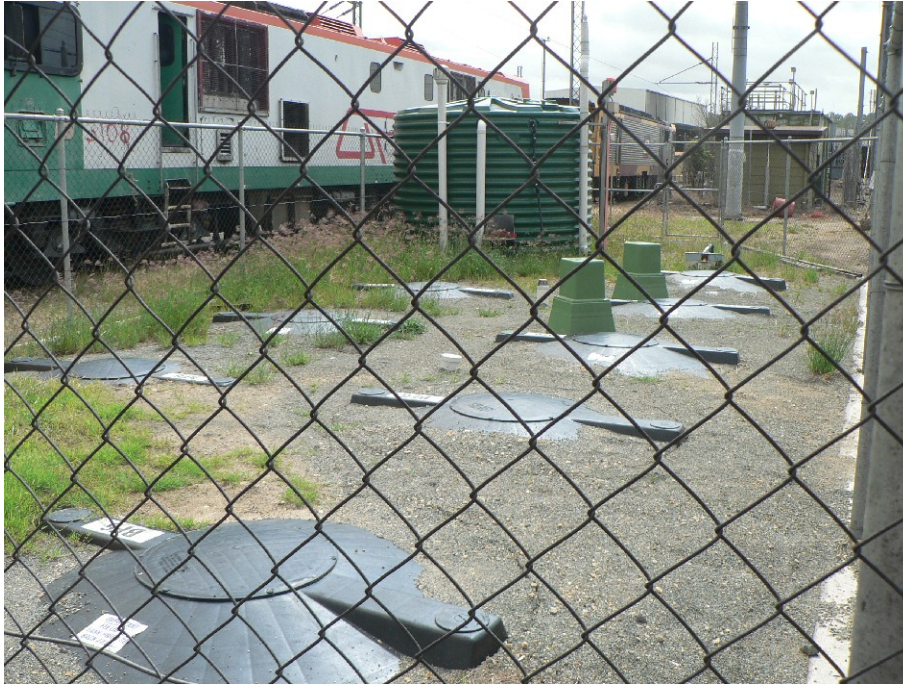
Photo 11.1 Jilalan sewage treatment plant
