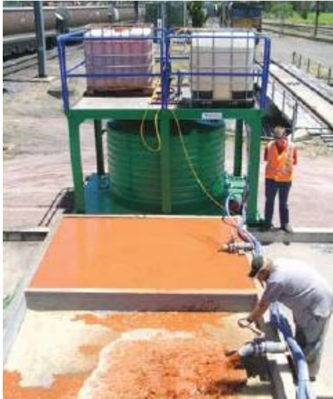
Photo 11.3 ViroFlow trade waste treatment system
