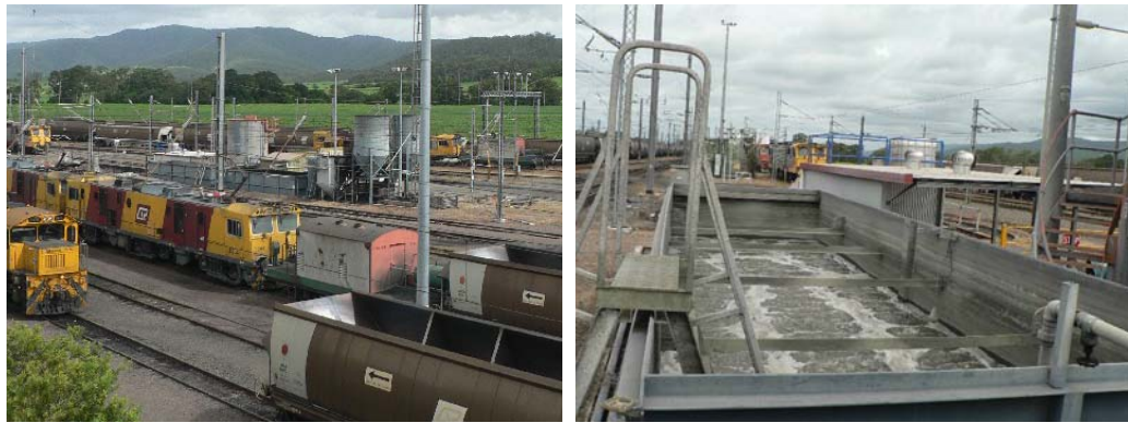
Photo 11.2 Pollution treatment plant (PTP)
