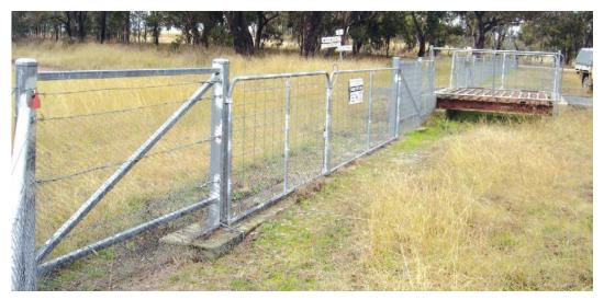
Photograph 3.1 Example of a rabbit-proof fence design with a gate trap
