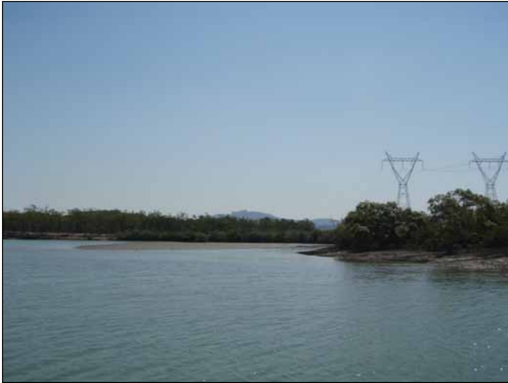
Figure 7 Seawater intake location, looking north, showing exposed mudflats, anabranch (to the right) and eroded bank (top left)
