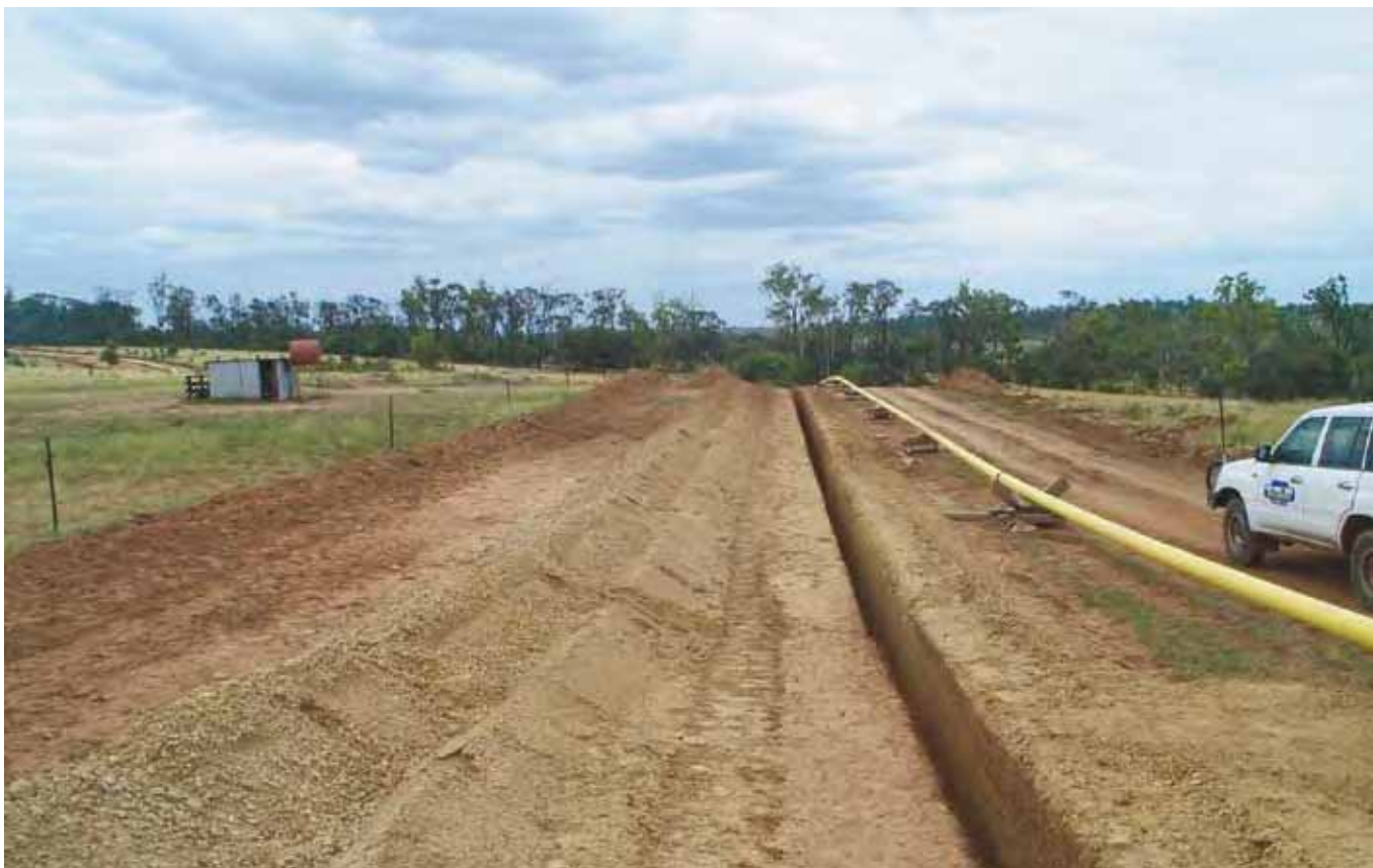
Pipeline installation at Scotia. Preservation of topsoil (far left), separation of soil types (left of trench) and protection of soils from vehicle movement can be seen.
