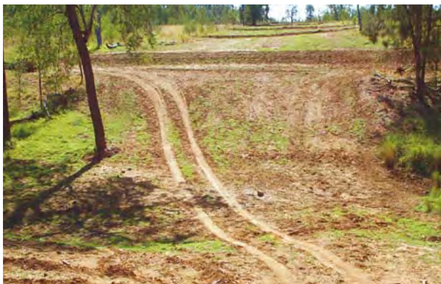
Creek rehabilitation at Scotia. Contour banks (at back) installed to divert water from pipeline route and minimise erosion
