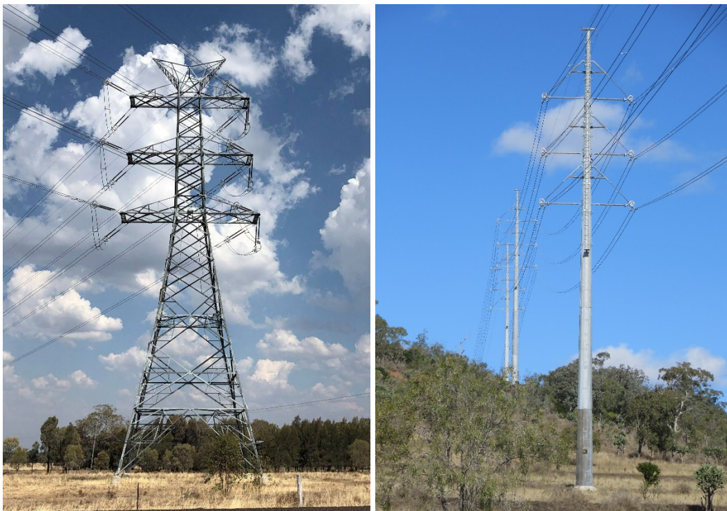
Plate 2-1 Typical 330kV double circuit steel lattice transmission tower (left) and typical 330 kV double circuit monopole (right)
