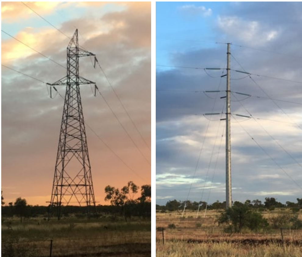
Plate 2-2 Typical 220 kV single circuit lattice transmission tower (left) and typical 220 kV single circuit monopole structure (right)
