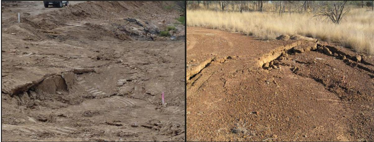
**Figure 40. Heaving and Buckling.**
