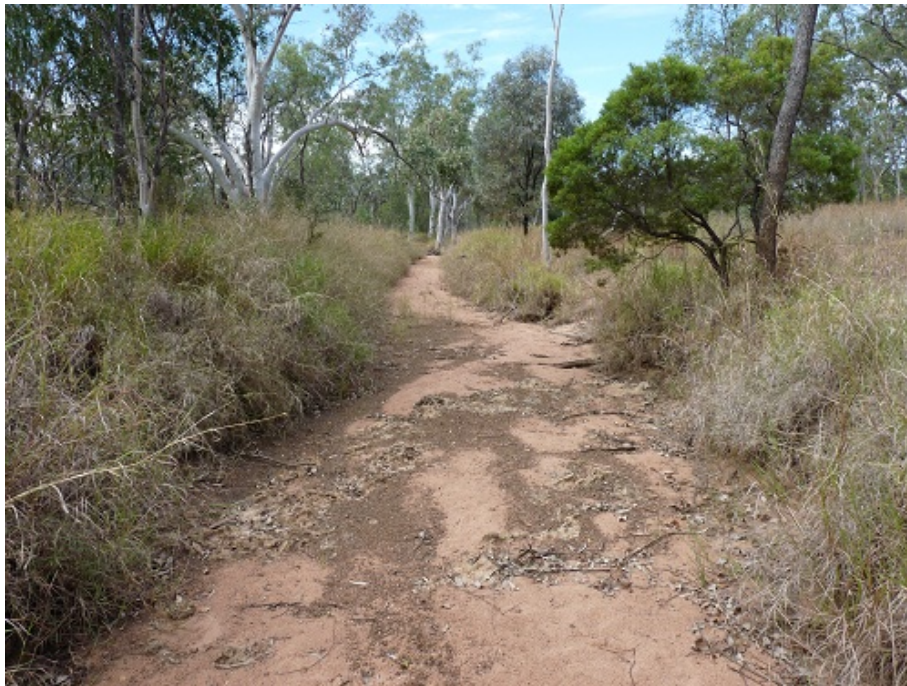
Plate 5 Upstream view of a stable channelised fill section exhibiting evidence of sand accumulation from the release of sediment from ongoing upstream incision processes
