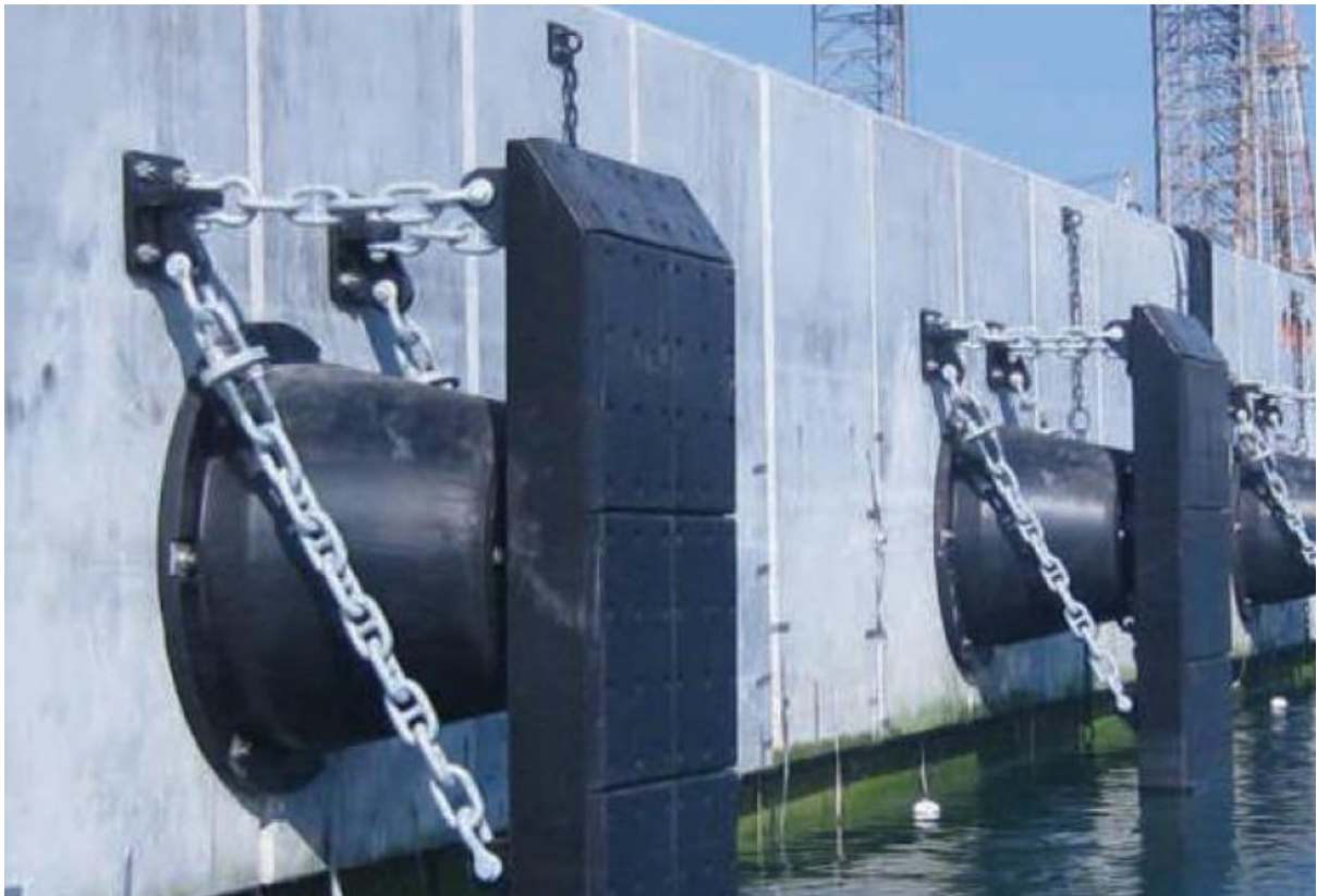
Figure 31. Indicative view of an installation of 'Super-Cone Fenders (at Bahrain) (Source: Ports North).
