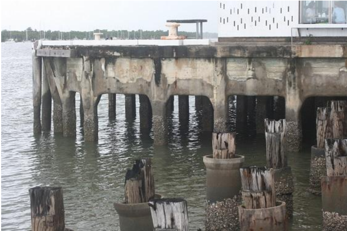
Figure 20. The reinforced concrete structure is apparent at the north end of Wharf 1.
