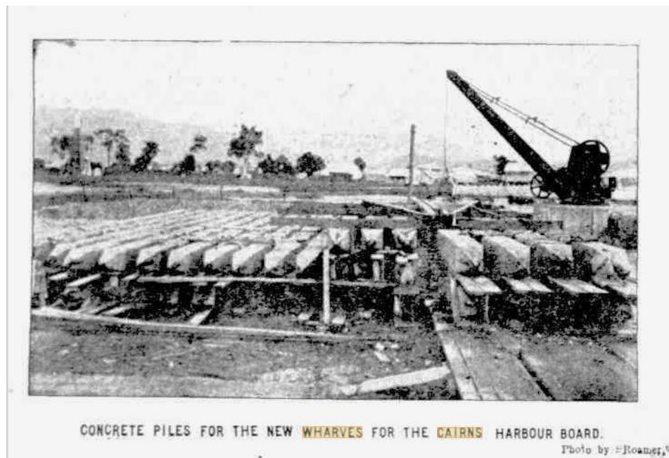
Figure 12. Photograph of the Concrete Piles for the Cairns Harbour Board, published in 'The Week', Friday, 30 December, 1910. (Source: Trove)
