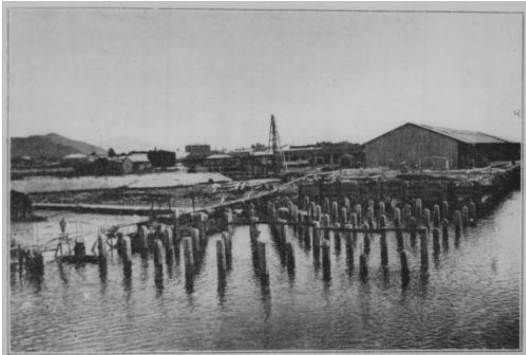
Figure 15. New section of reinforced concrete wharf (Wharf 5) under construction at Cairns, circa 1923. (Source: SLQ #199171)
