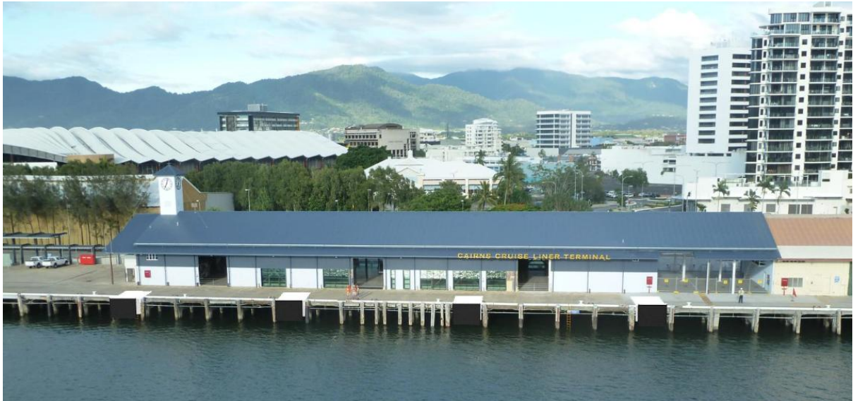
Figure 30. Generated image of the proposed new berthing dolphins inserted into the wharf deck (visible as white/black patches along the front of the wharf. (Source: Ports North)
