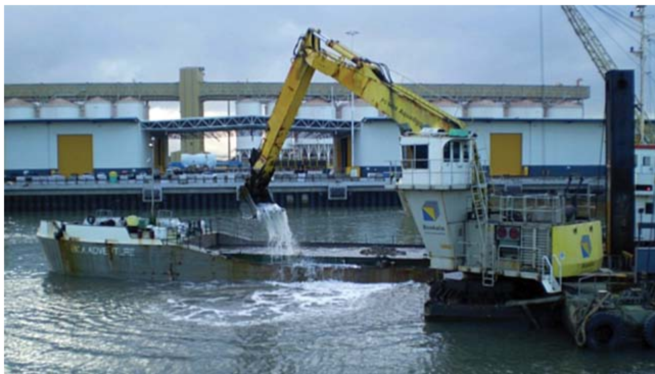
Figure C3.6.1a BHD Dredging and Loading into Hopper Barge
