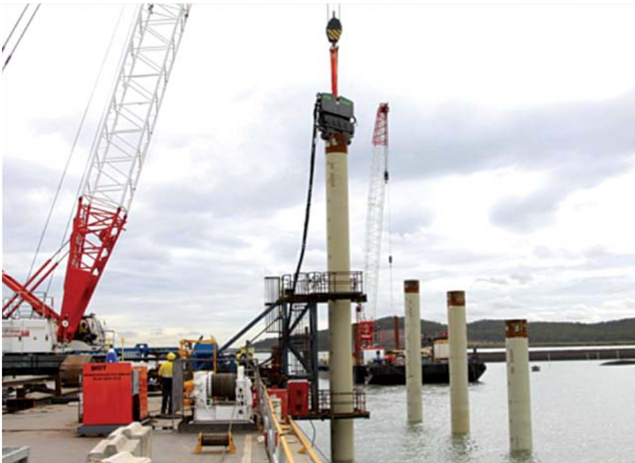
Figure C3.6.2a Example of a Pile Driving Barge
