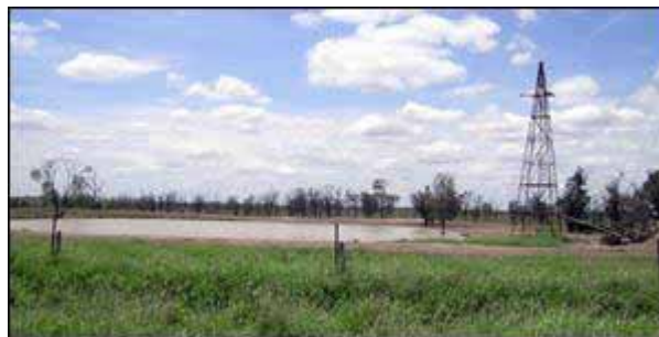
Figure 15.4 South-east view - Damaged windmill and one of two nearby dams.
