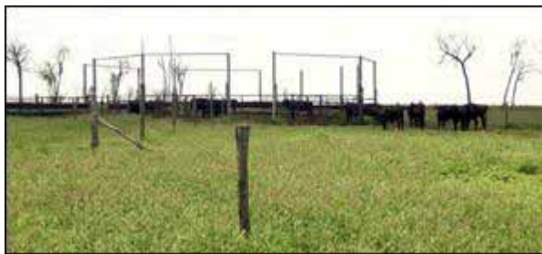
Figure 15.5 Southern view - Timber and steel cattle yards and trough.
