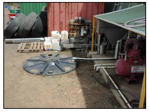
Plate 4 In-ground Waste Oily Water/sediment tank - Kalari Yard
