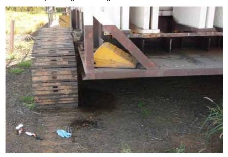
Plate 30 Oily stain under Transformer TSS01 – Peak Downs Mine
