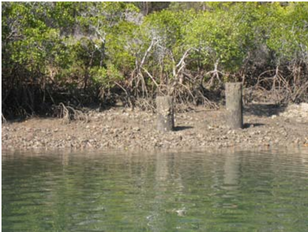
Plate 3 Jetty remnants on southern bank of Graham Creek.
